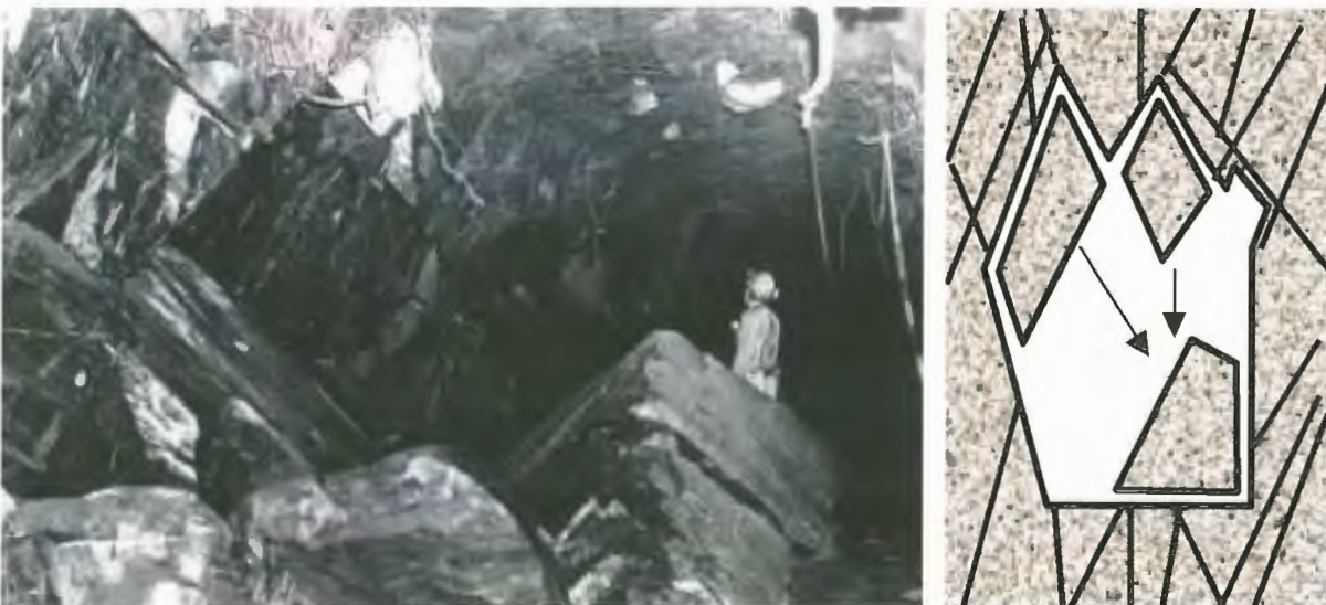
Figure 45: Photograph and sketch demonstrating observable signs of low stress failure (Photograph courtesy of Mount Isa Mines Ltd)
