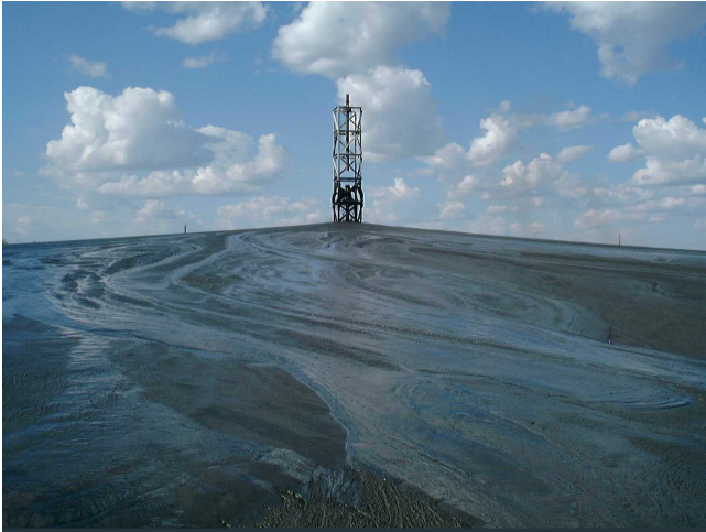
FIGURE 1.2 Bulyanhulu – an example of high-density thickened tailings deposition
