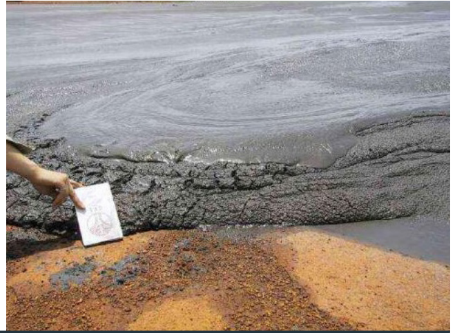
FIGURE 1.2 Bulyanhulu – an example of high-density thickened tailings deposition
