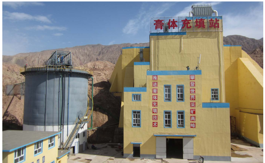
Figure 1 The paste backfill station at Jiashi Tonghui Copper Mine
