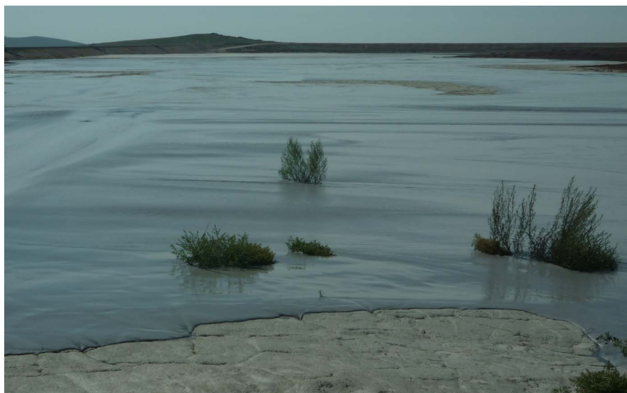
Figure 2 Paste flow in the Wushan Copper Mine tailings pond
