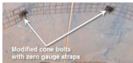
Figure 4 Final product of burst-resistant (dynamic) support system used in one of the drill sills at Copper Cliff Mine
