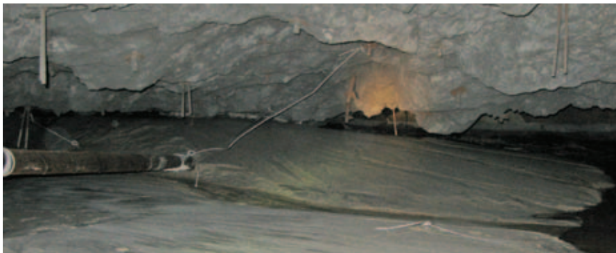
Tight filling in progress in a stope
