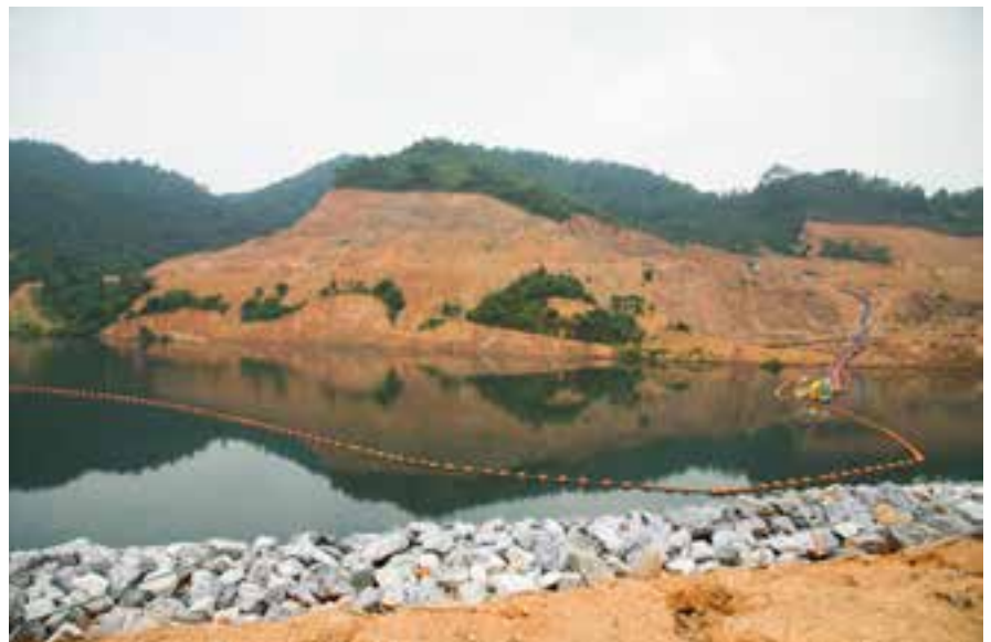
Designers, owners and operators of TSFs face ongoing challenges in meeting the needs to safely store large volumes of tailings into the future
